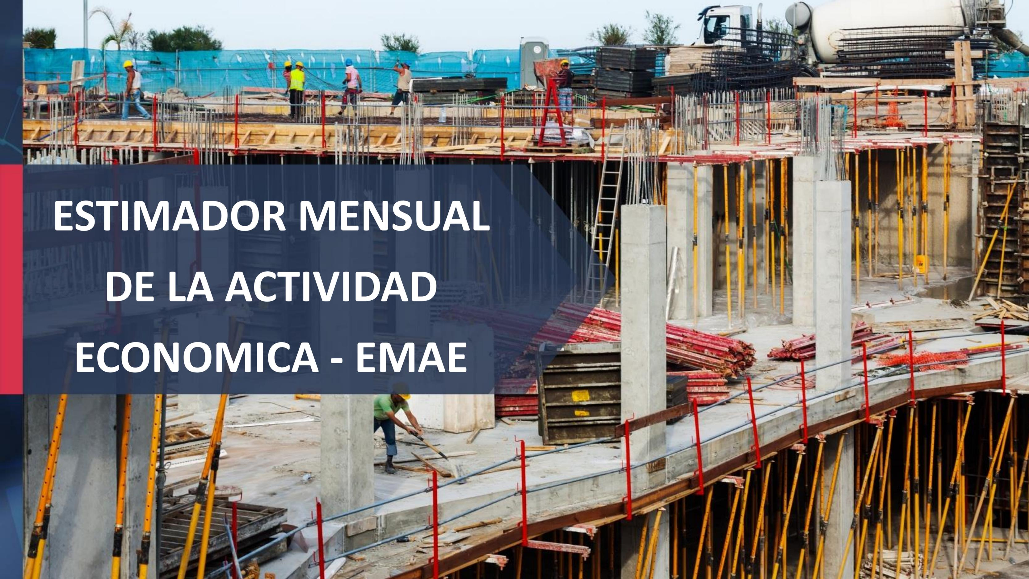
A large-scale construction site showing the preparation of a concrete slab. The scene is filled with a dense network of steel reinforcement bars (rebar) and wooden formwork. Several workers in safety gear are visible on the upper levels of the structure. In the background, a concrete mixer truck is parked. The foreground shows a worker in a green shirt and blue pants using a tool on the ground level. The overall atmosphere is one of active construction.
